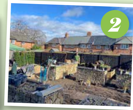
2 GO, GO, GABIONS! Painstakingly filled with stones by the landscapers, they form a screen in front of the allotment garden.
