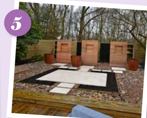
ROUNDED PEBBLES of different sizes cover the ground surface, the steel planters are positioned, and the decking is finished.
