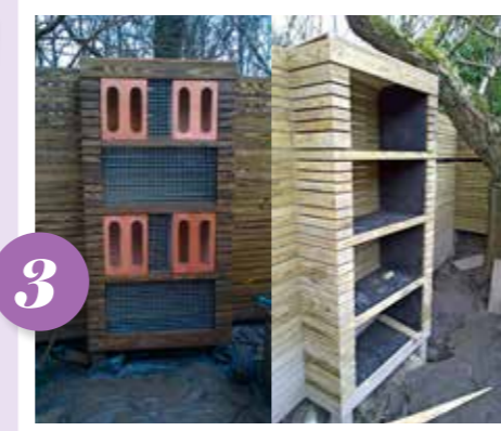
THE BUG HOUSE is made with wire grids to hold tree bark, straw and paper; the log store is constructed; and a weedproof membrane laid.
