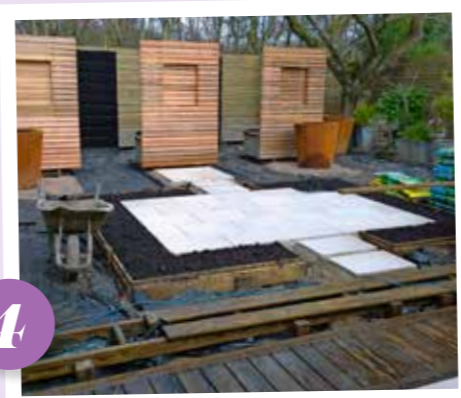
THE PAVING IS DOWN , the screens are in, and topsoil and gravel added. Work begins on the decking outside the bifold doors.
