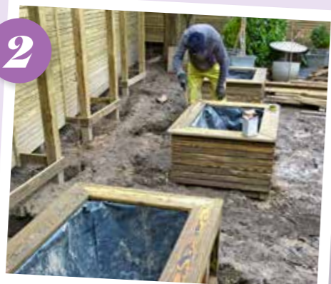
THE PLANTERS ARE BUILT from hard southern pine, lined with plastic, and the framework for the living walls is created.
