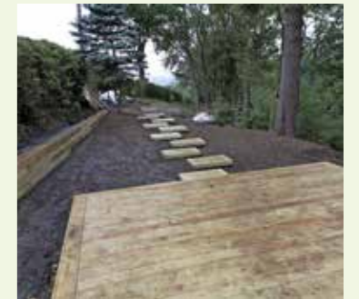
A platform, staggered stepping-stone pads and a weed-stopping wall are built from American pine.
